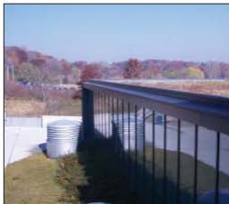
Green Roof, RAWC Building
