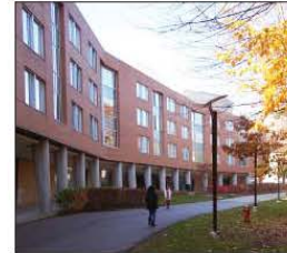
Erindale Hall, north elevation
