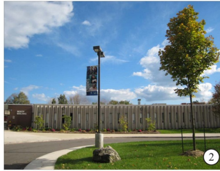
Drop-off loop in front of North Building
