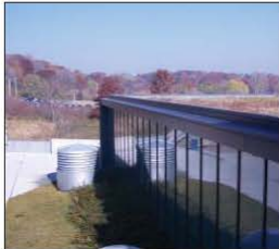
Green Roof, RAWC Building
