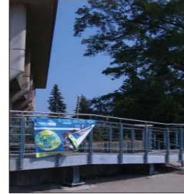
Accessible Entry, Davis Building
