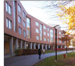
Erindale Hall, north elevation
