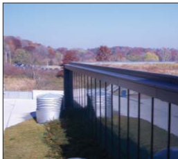
Green Roof, RAWC Building
