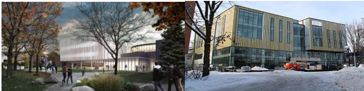
Rendering of Innovation Complex courtesy of Moriyama & Teshima North Building Reconstruction – “Deerfield Hall” Photo by Gareth Trickey Architects and PCL Constructors Canada Inc.
