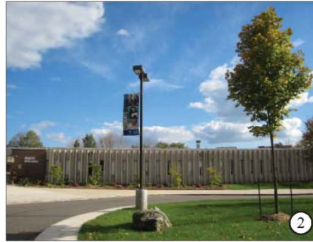
Drop-off loop in front of North Building
