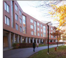
Erindale Hall, north elevation
