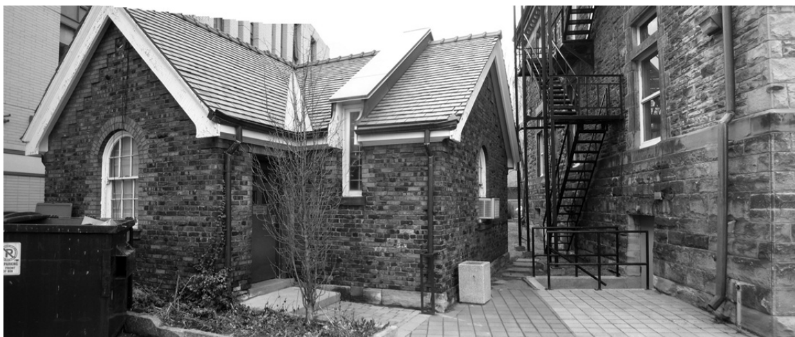
Registrar's office/Transit House, located on the west side of main building (2009)
