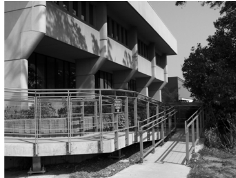
Existing exterior view – SW Entrance
