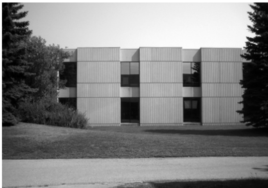
Existing exterior view – NW Elevation
