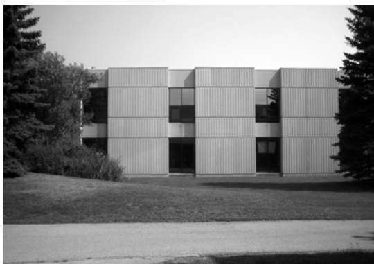
Existing exterior view – NW Elevation
