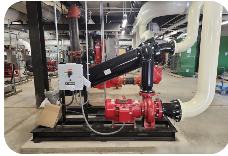
Chiller plant optimization
