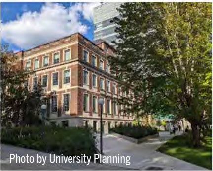
2024 | FitzGerald Building Revitalization
