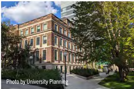
2024 | FitzGerald Building Revitalization
