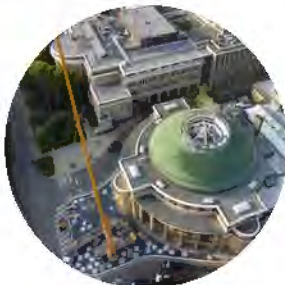
Condition of Campus Facilities
