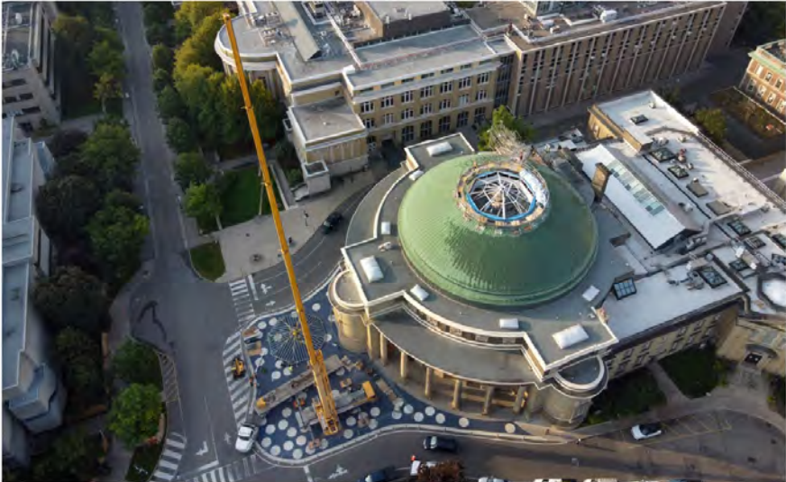
Condition of Campus Facilities
