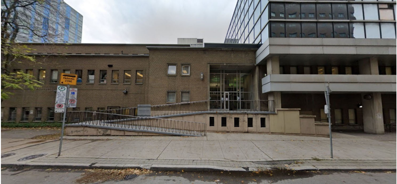
Photo 03_Elm Street Patient Entrance and Exterior Ramp
