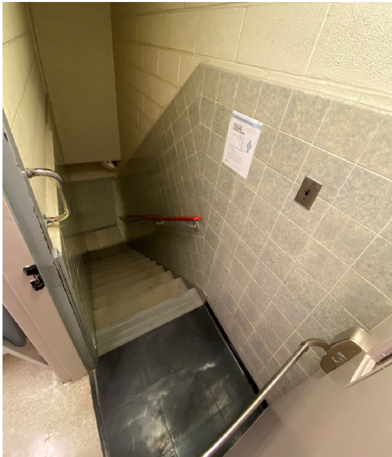
Photo 04_124 Existing Egress Stair connecting Clinic 1 to 3 rd Floor
