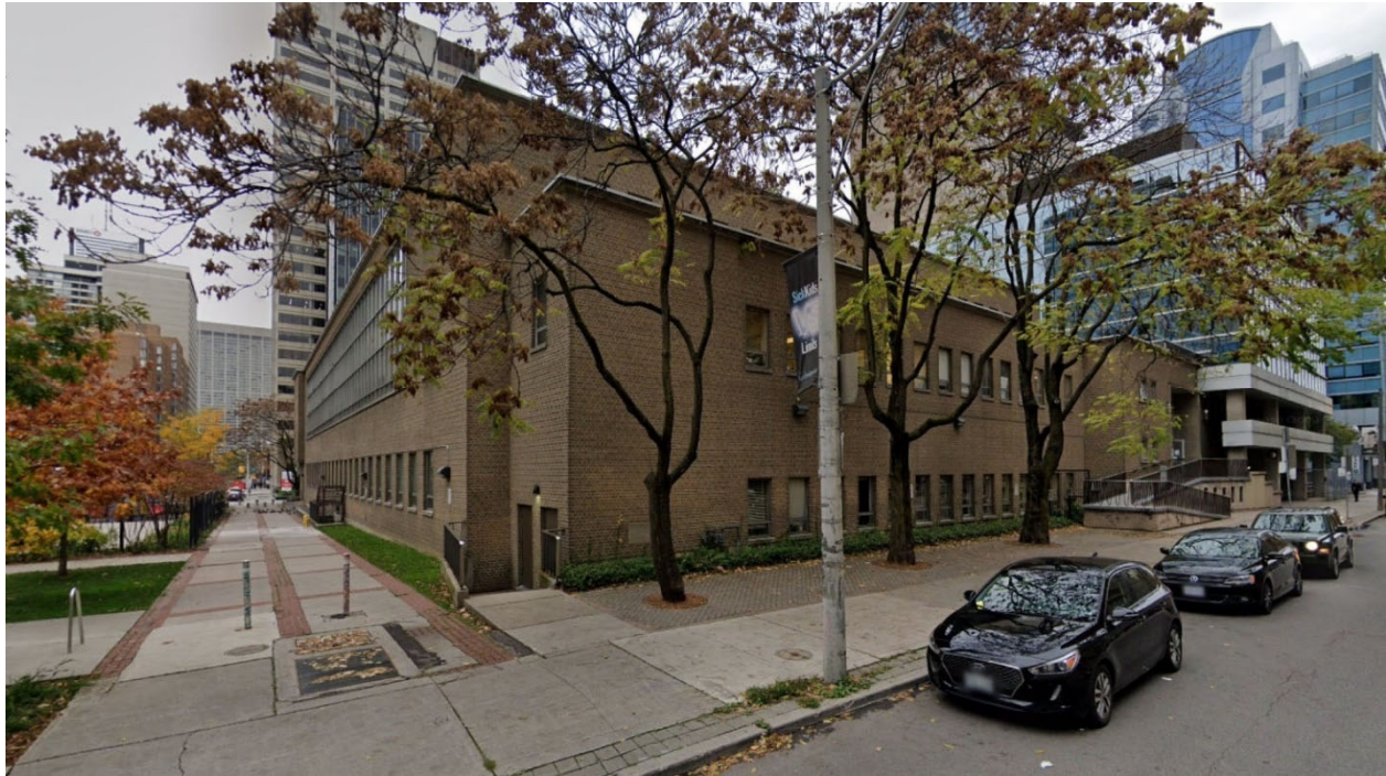
Photo 07_Existing Second and Third Floor Windows at East and North Façade
