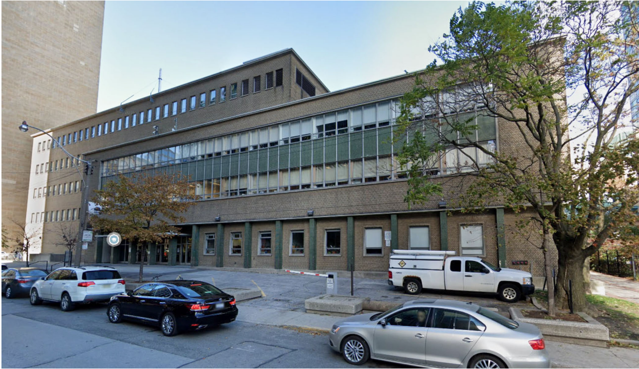
Photo 01_124 Edward Street Building 065 South Elevation
