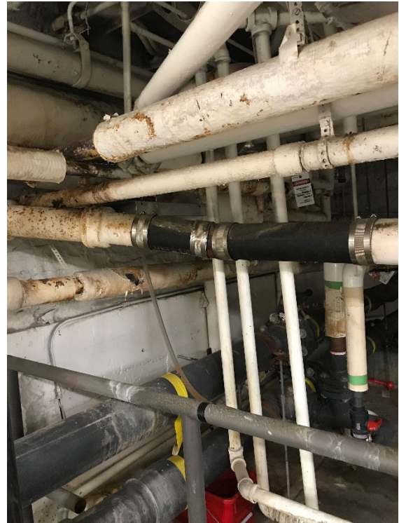
Pool room pipes – old and new
