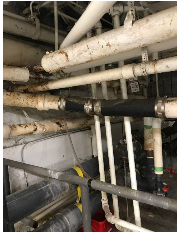
Pool room pipes – old and new
