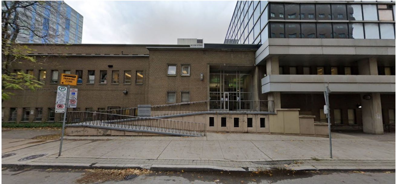
Photo 03_Elm Street Patient Entrance and Exterior Ramp
