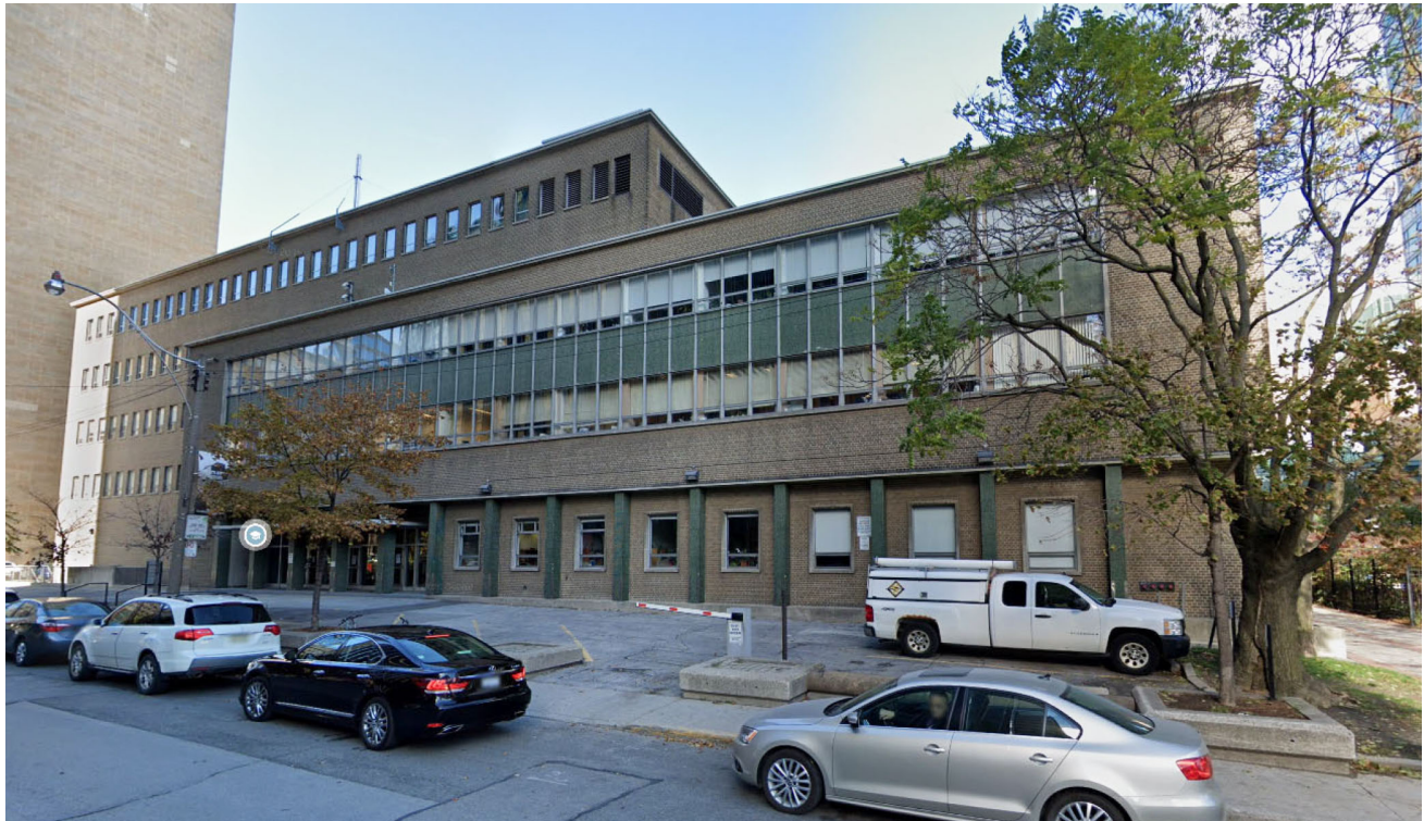
Photo 01_124 Edward Street Building 065 South Elevation
