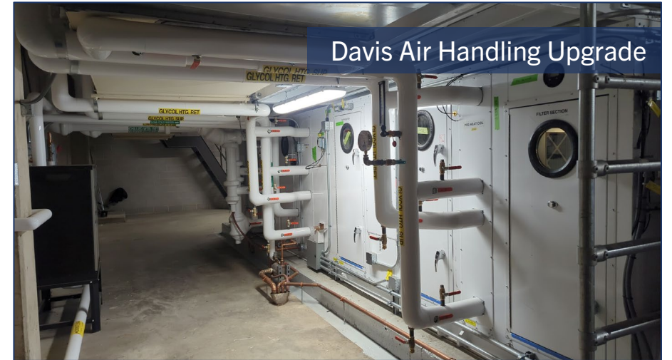
Master Services Upgrades
