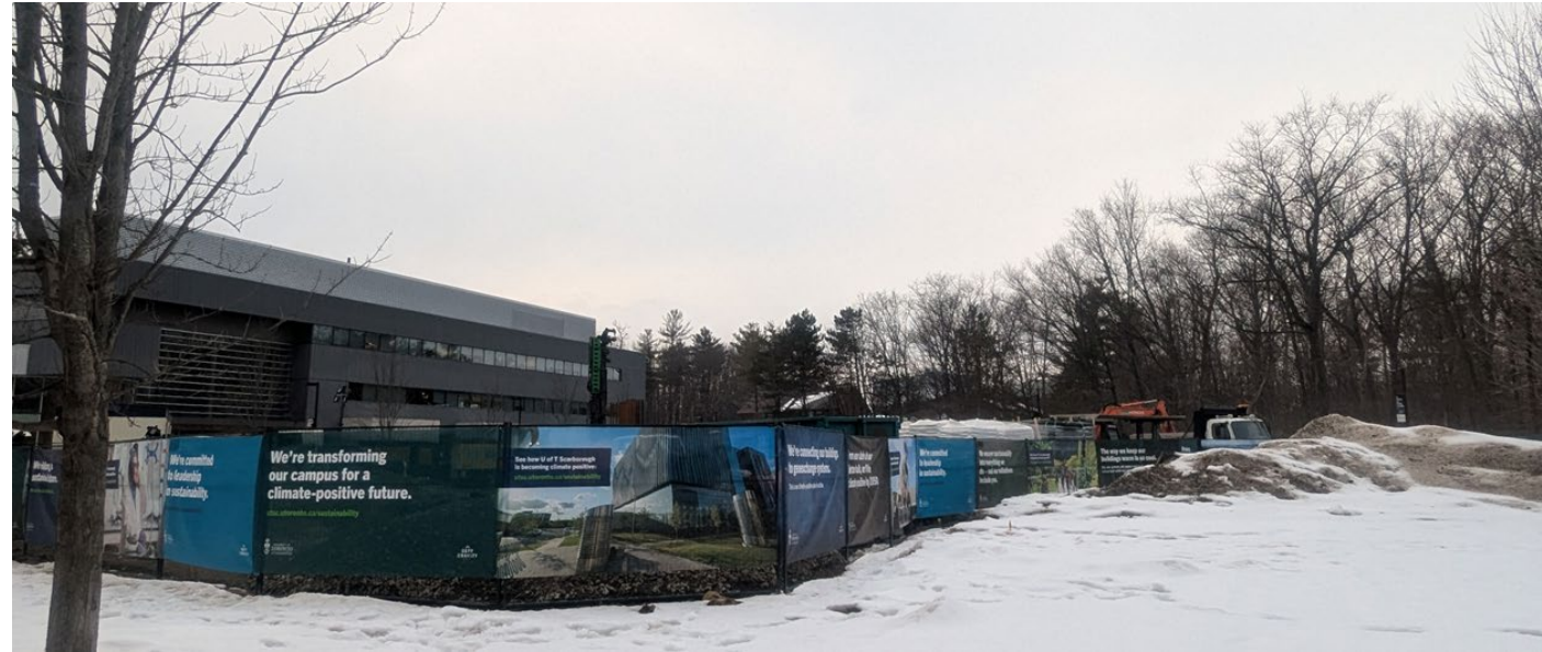
Image caption (above): Current geo-exchange drilling in S-Wing Quad (Winter – Spring 2026)
