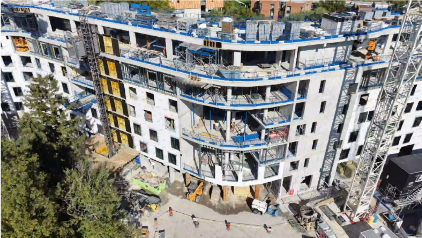
Progress on construction as of October 9, 2025
