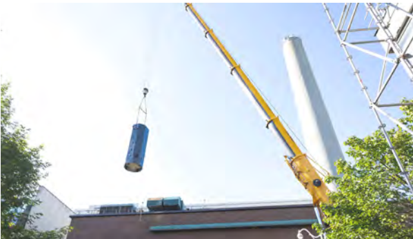
A new electric boiler being lifted into the Central Steam Plant (photo by Johnny Guatto)
