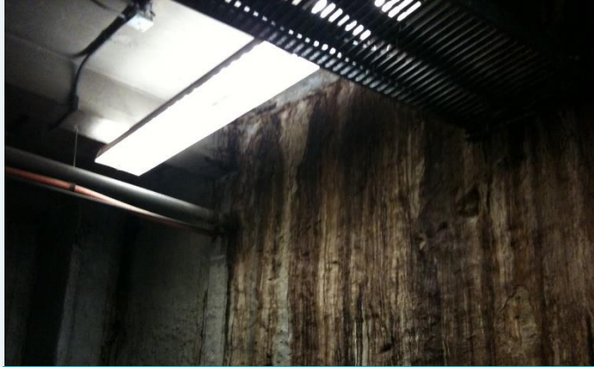
Main Electrical Room Water Infiltration
