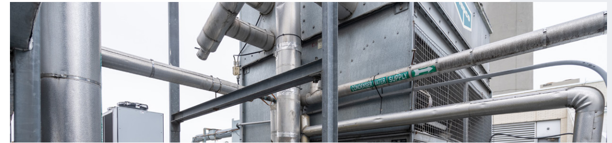
Photo: Infrastructure at BCIT (Donglin Que)
