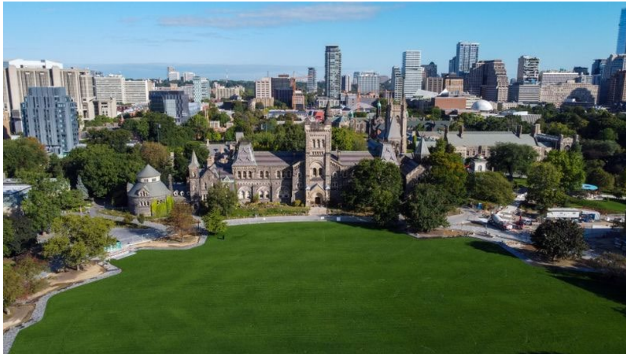
Completion of the public green above the geothermal exchange. Photo by David Lee.
