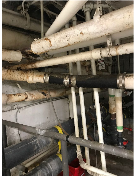
Pool room pipes – old and new
