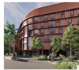
Phase IX Residence UTM
