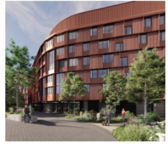
Phase IX Residence UTM
