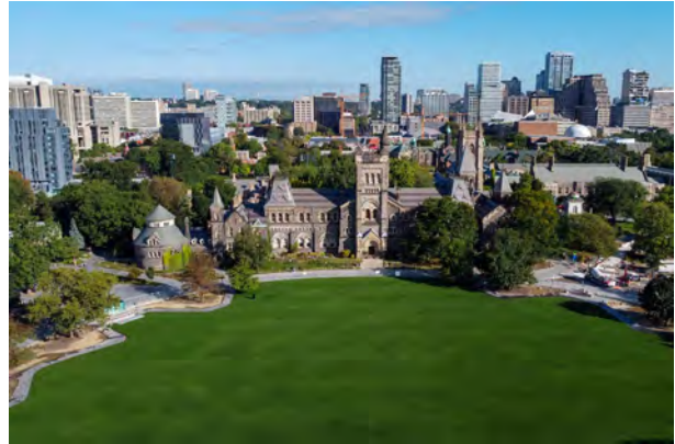
After: Completion of the public green above the geothermal exchange. Photo by David Lee.
