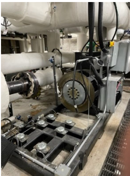
Figure 8: Removed Back Pressure Turbine in CSP
