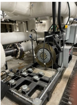
Figure 8: Removed Back Pressure Turbine in CSP
