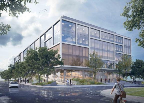
UTSC Instructional Centre 2; CEBRA / ZAS Architects + Interiors
