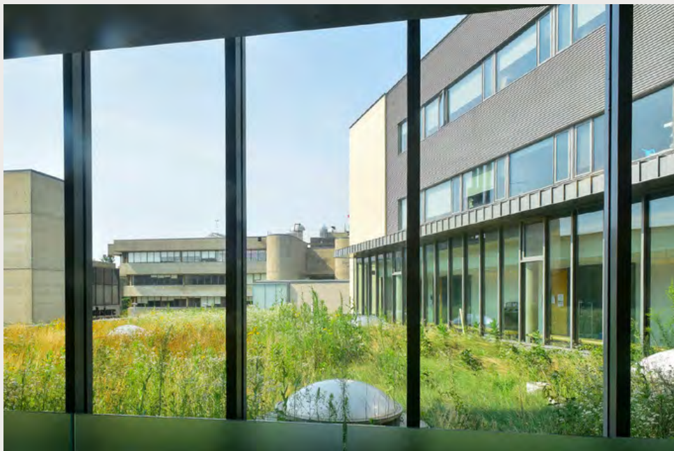
UTSC green roof. Photo credit: Ken Jones.
