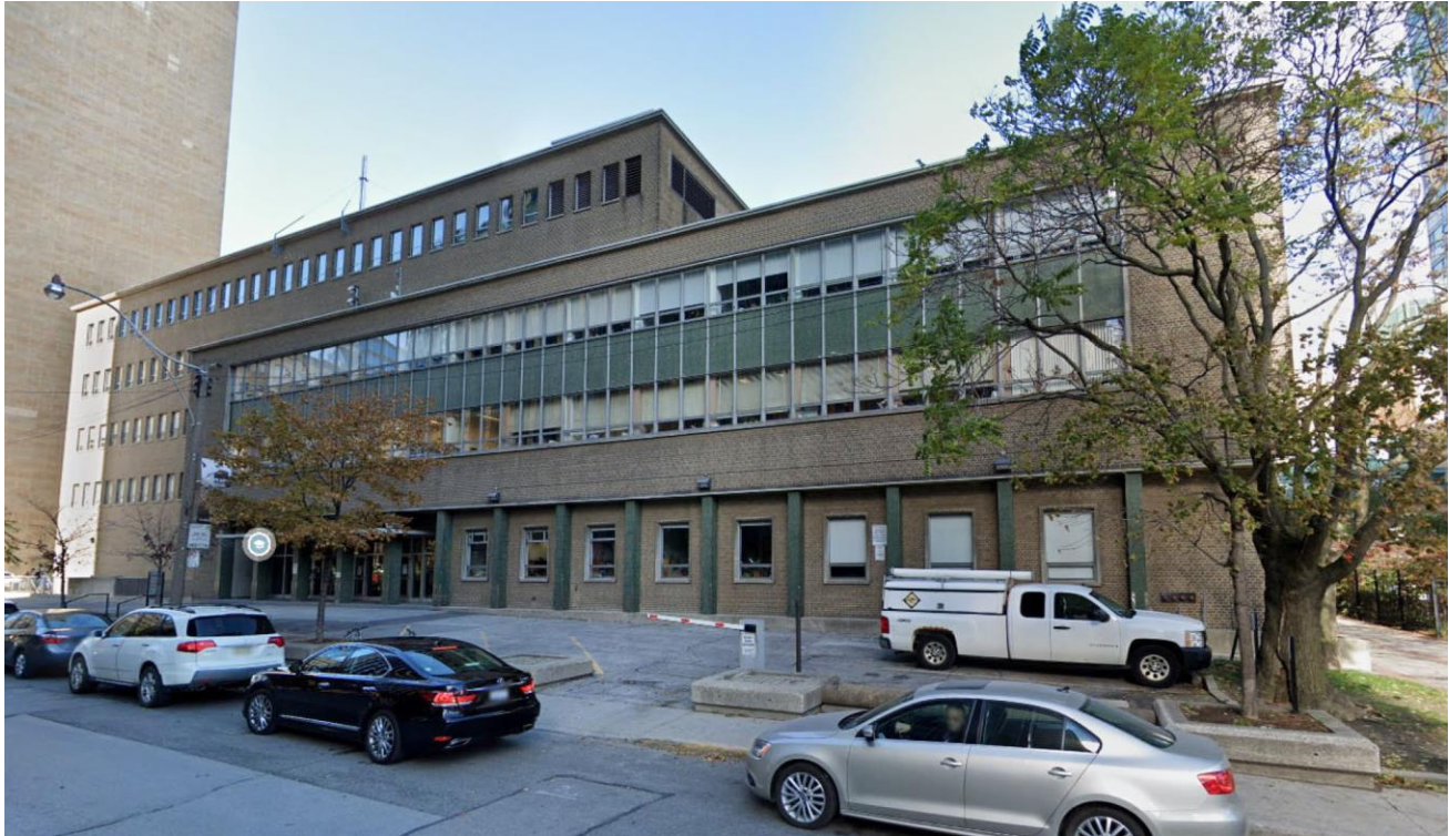
124 Edward Street Building 065 South Elevation
