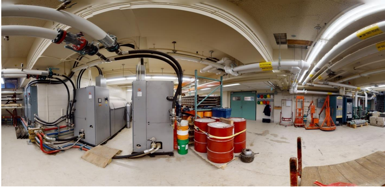
EXISTING STRUCTURAL LAB (GB16 east panorama – inc. Hydraulic Pumps)
