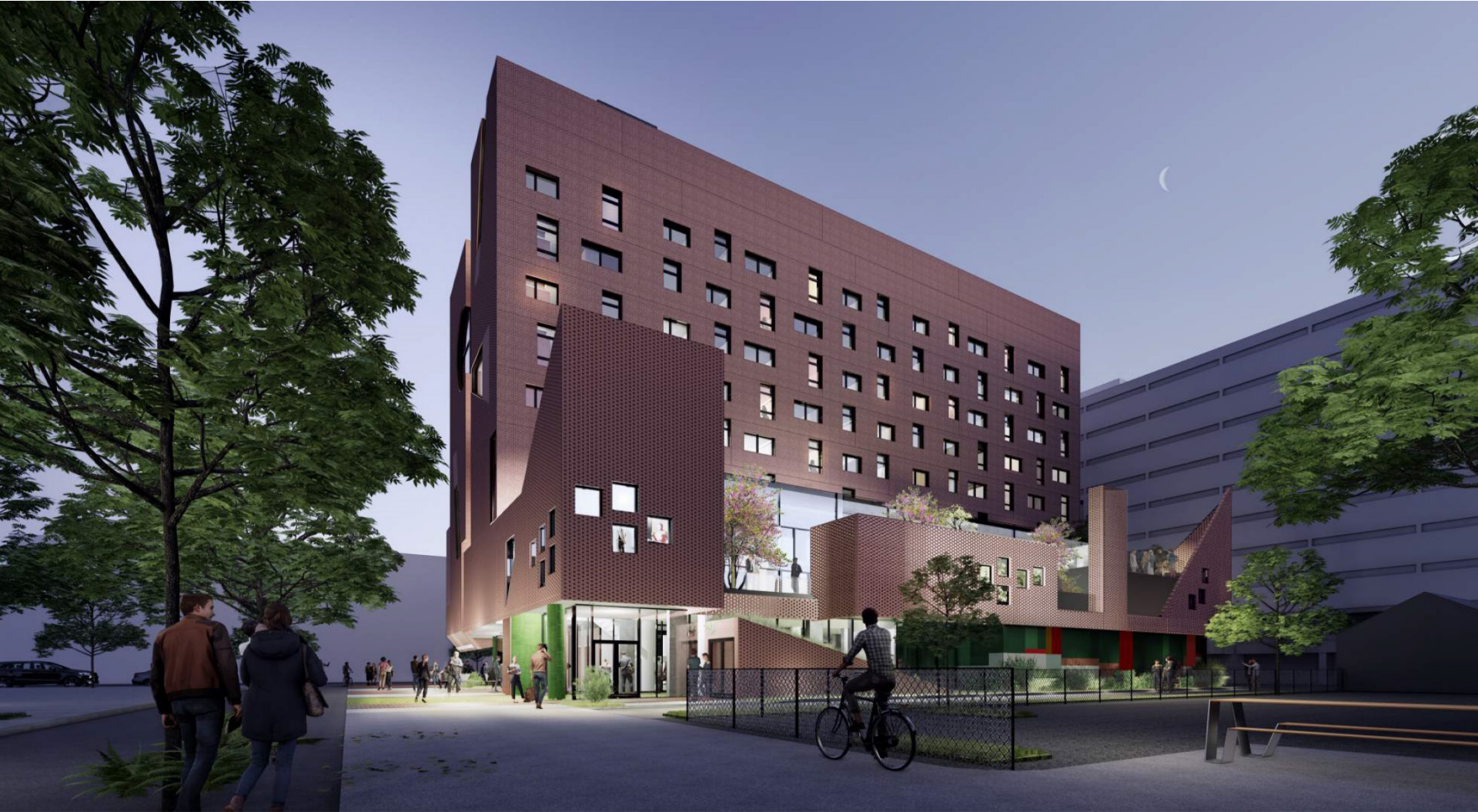
View from the North-East
