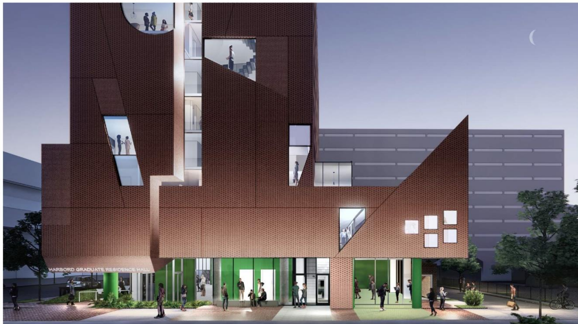
Figure 21 – View of East Façade – Lower Floors: Image Courtesy of Michael Maltzan Architects / architects Alliance
