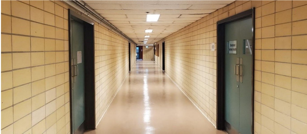
EXISTING HALLWAY 19K (looking west)
