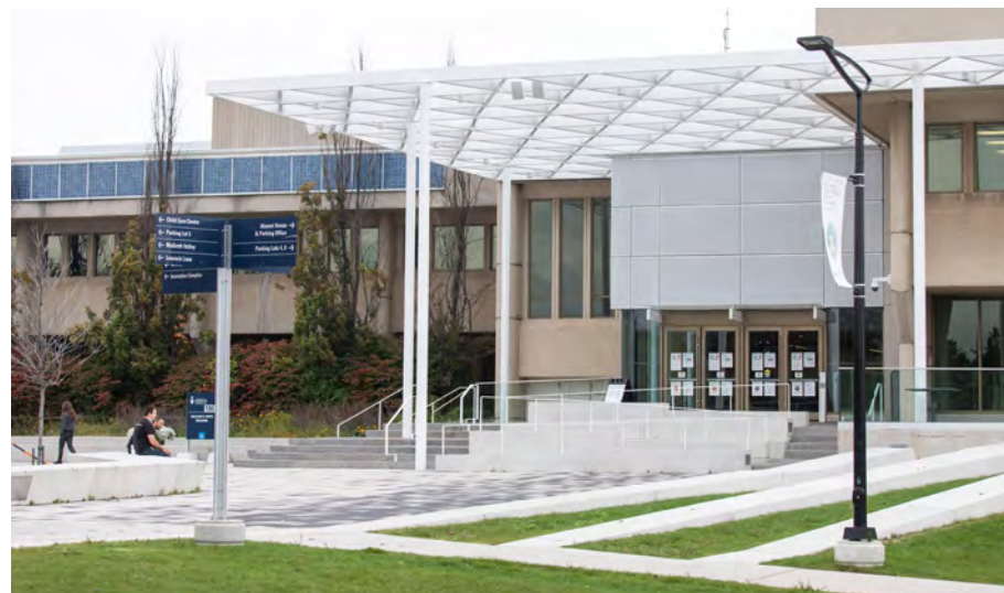
William G. Davis Building expansion
