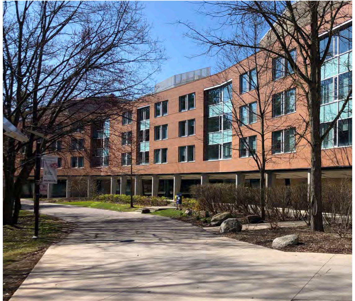
View of the existing Five Minute Walk pedestrian street adjacent to Erindale Hall Residence.
