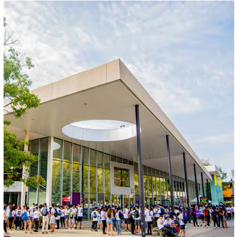
The redesigned Residence Road can be used for university events by closing off a portion of the street.
