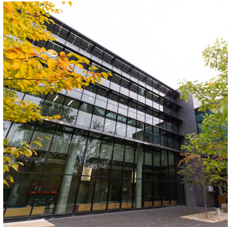
Buildings should consider innovative design to reduce heat gain, such as the brise soleil incorporated into the campus' Instructional Centre.
