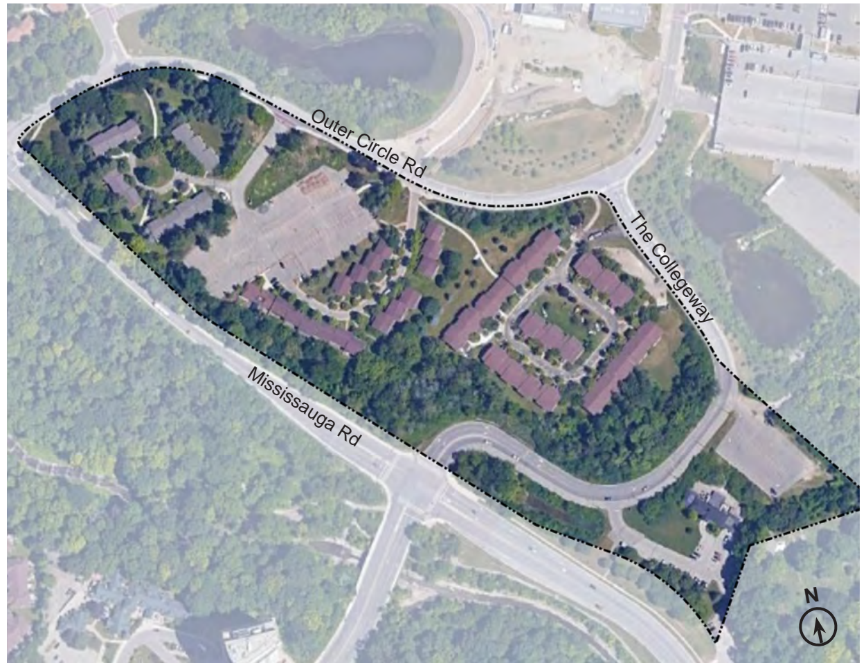
Aerial view of the existing Campus South Precinct.
