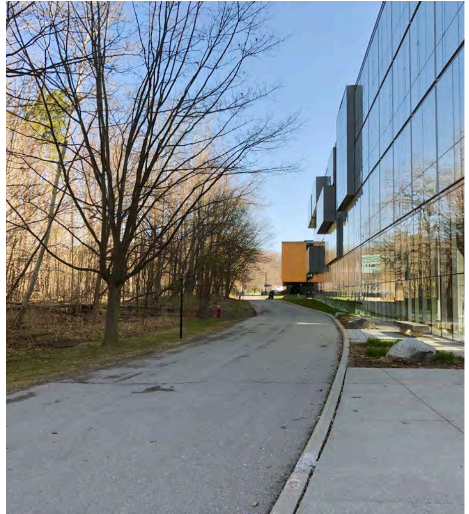
View of Middle Road adjacent to the CCT Building, looking east.
