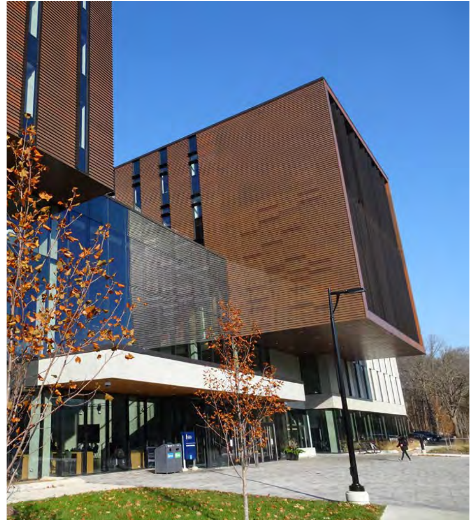
View of the Maanjiwe nendamowinan building within the Core Campus Precinct.
