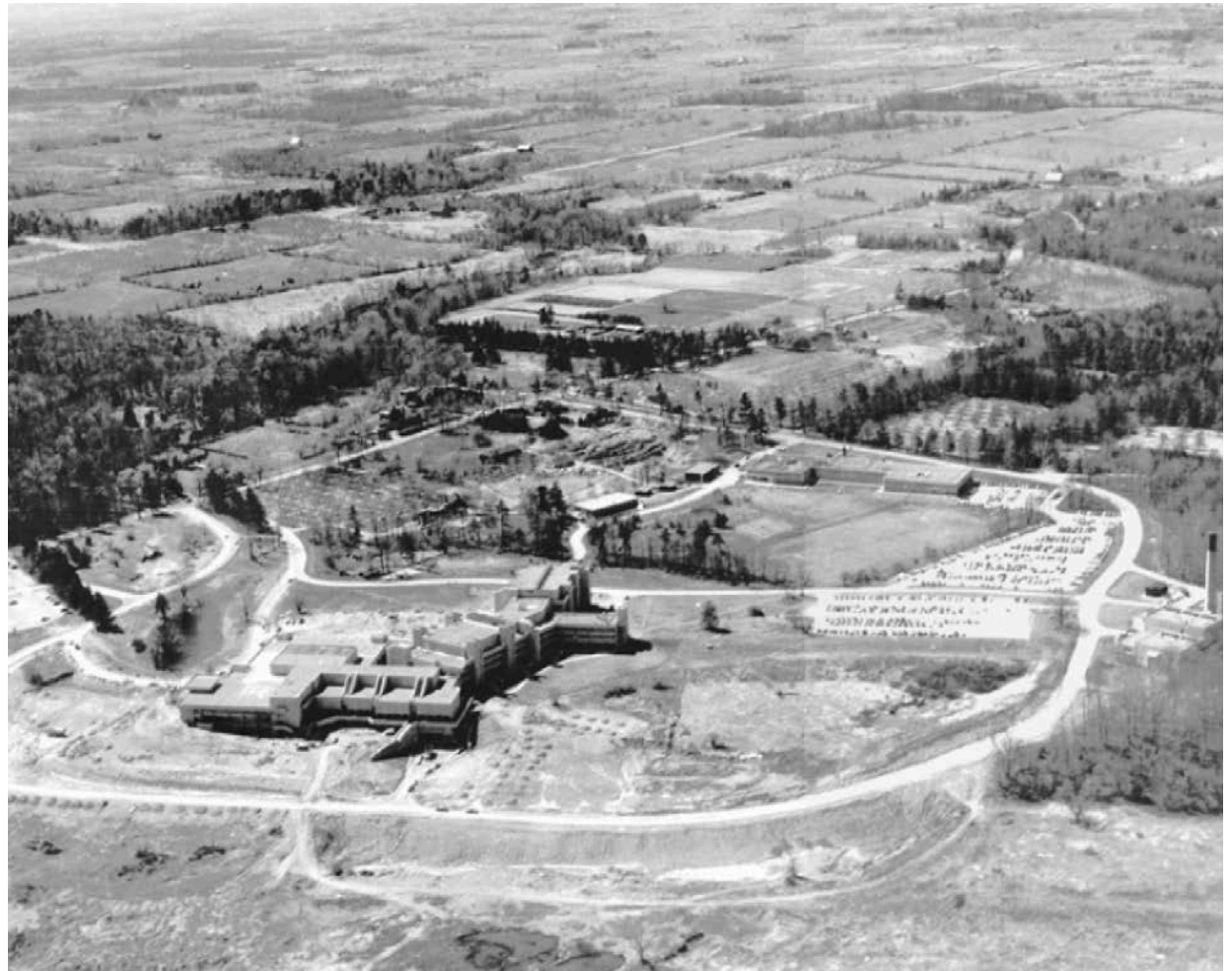
Early campus development (circa 1972) included the South Building, the current theatre building, and the former North Building, bounded by Outer Circle Road.
