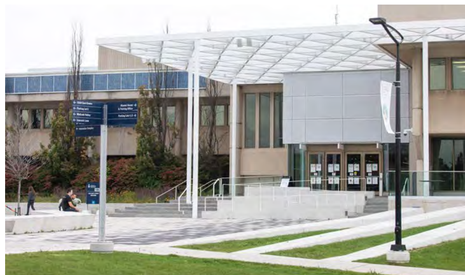
William G. Davis Building expansion
