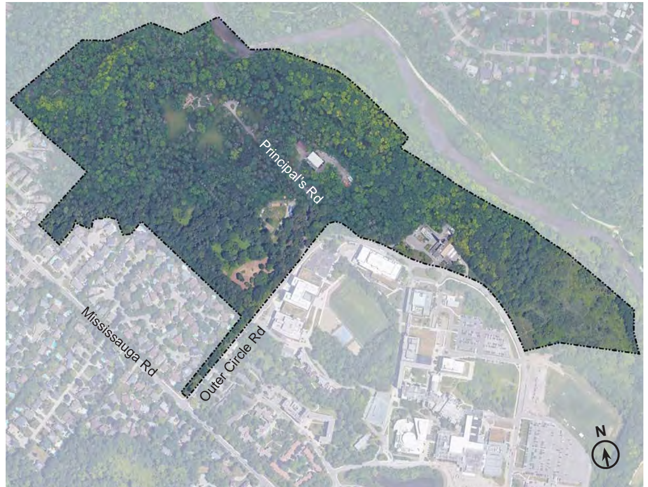
Aerial view of the existing Forest Precinct.
