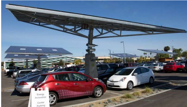
Roof-mounted photovoltaic panel example
