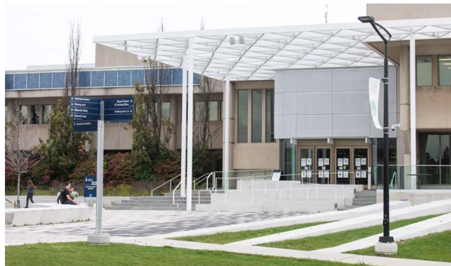
William G. Davis Building expansion
