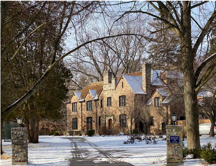
Lislehurst is UTM's principal's residence, a designated heritage building designed in the Tudor Revival style.
