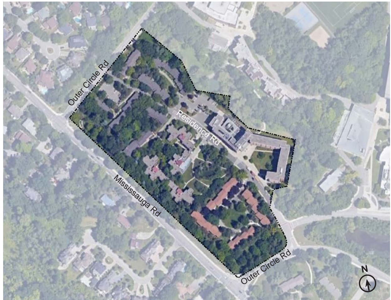
Aerial view of the existing Campus Southwest Precinct.
