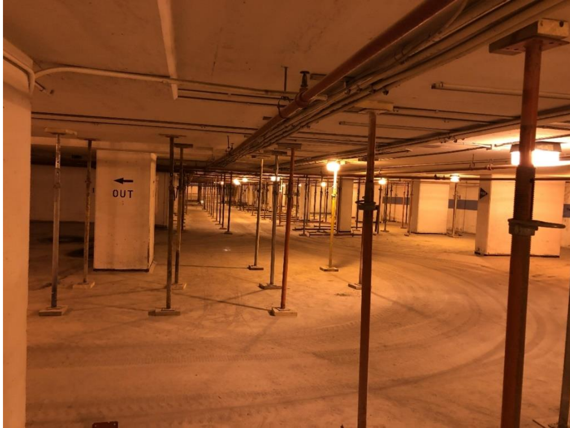
CHESTNUT RESIDENCE PARKING GARAGE RENOVATION $2.3M
