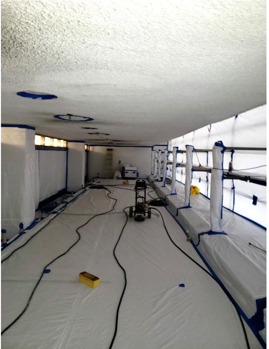
CLARA BENSON POOL GALLERY RENOVATION $3.85M
