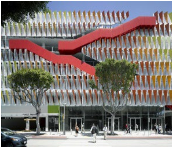
Parking Structure, City of Santa Monica, CA - Behnisch Arcitekten
