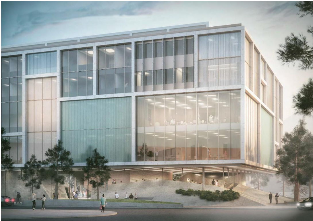
Rendered View of the North-East Corner of the IC-2 demonstrating the raised program space and printer's box façade approach (CEBRA/ZAS Architects)
