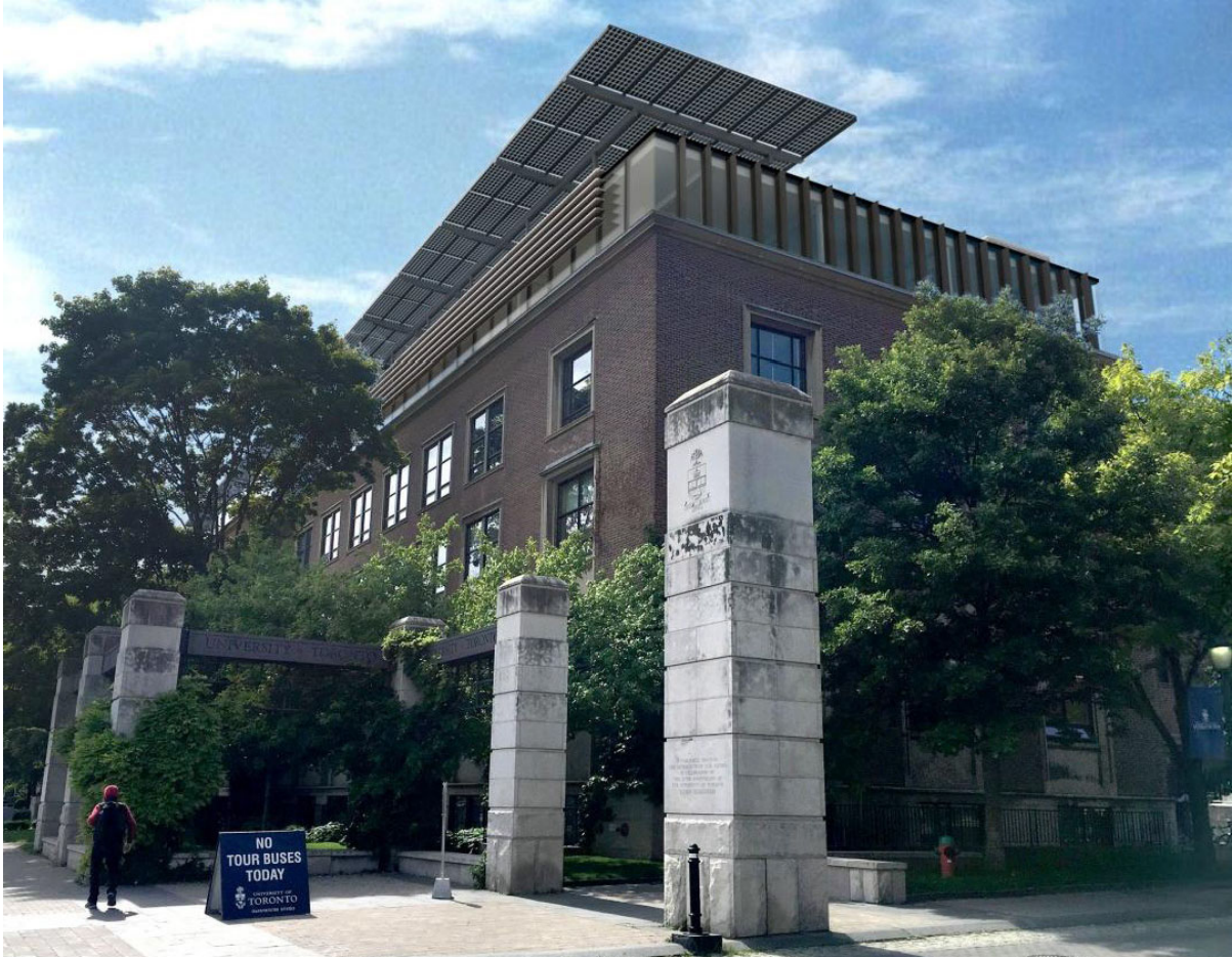
Proposed Sustainability Lab, Southeast corner of Wallberg Building at College St and King's College Road
