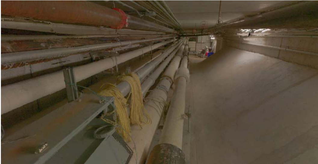
Figure 1 – LiDAR Scan of the Existing Steam Tunnel in Woodsworth College
