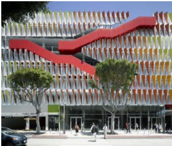
Parking Structure, City of Santa Monica, CA - Behnisch Architekten
