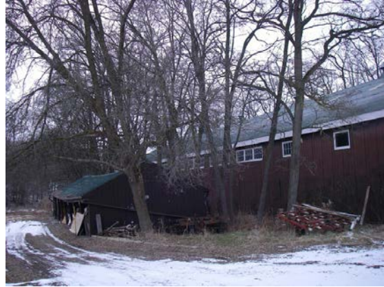
Out building at Arena Barn
